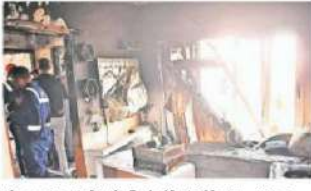
The apartment after the fire incident Friday. Anand/Anand
